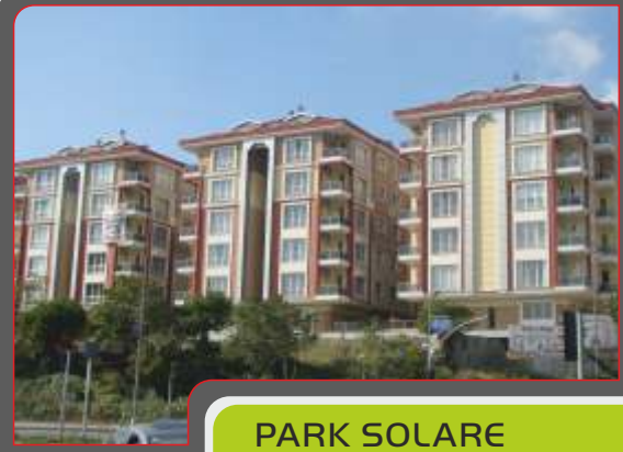
PARK SOLARE BAKIRKÖY
